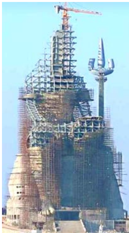
Fig. 11. Construction in progress
