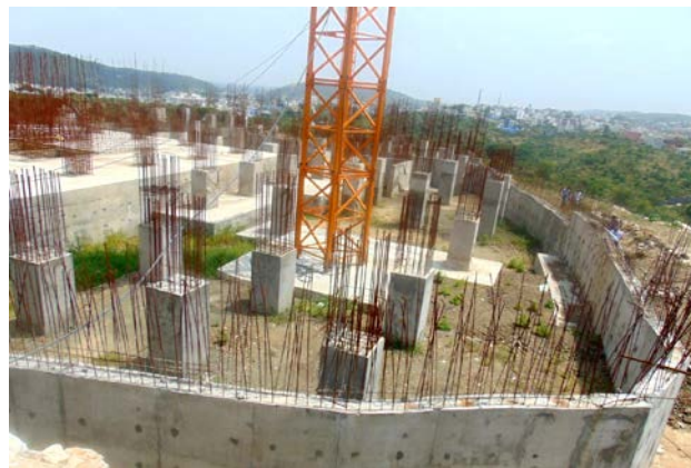
Fig. 9. Foundation construction in progress
