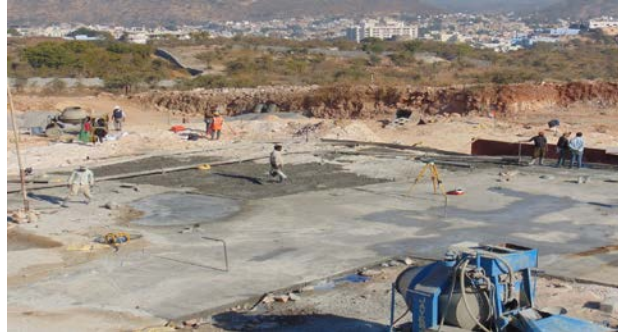
Fig. 8. Foundation level preparation
