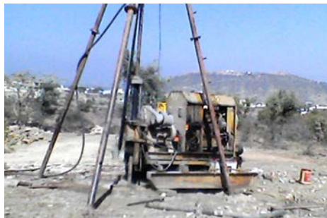
Fig. 5. Drilling in progress
